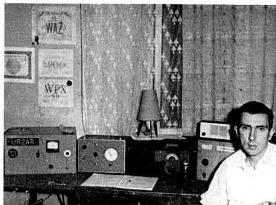
UR2AR, Enn Lohk, one of the leading s.s.b. stations in the USSR uses a three element quad with the home built equipment shown here.
